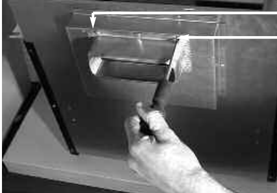
4 off Flue Spigot Fixing screws
